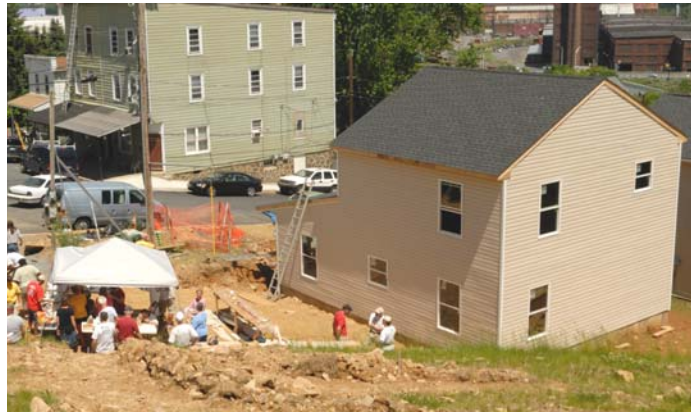
THE BLITZ-BUILD WAS COMPLETED TWO DAYS EARLY.
